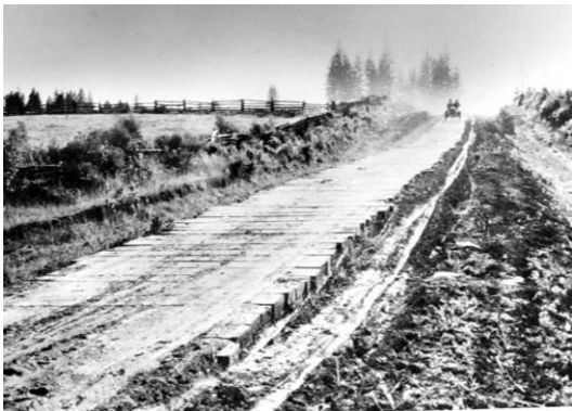
A Corduroy Road on the coast in 1917, at least you were out of the mud when it rained.
