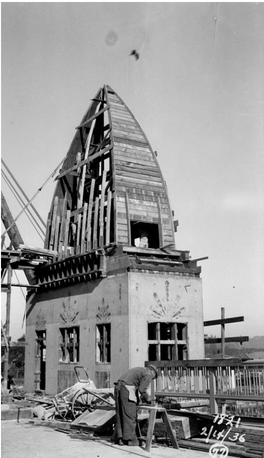
One of the four Bridge Towers under is construction.
