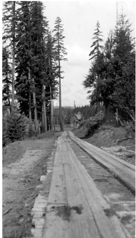
Looking south on a plank road south of Cannon Beach in the early twenties. Like the Corduroy Road it got you up out of the mud when it rained and it provided a lot smoother ride.
