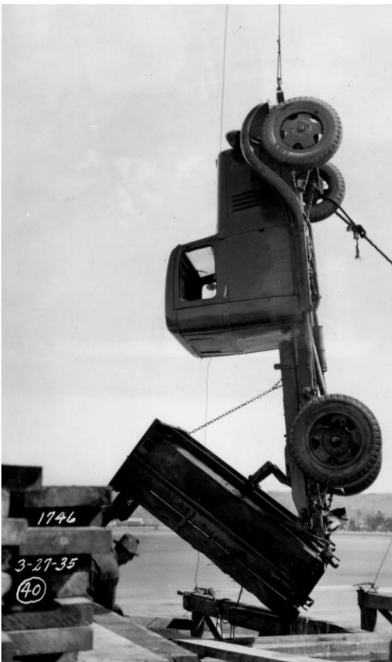
A wayward Ford construction truck is being fished out of Alsea Bay.
