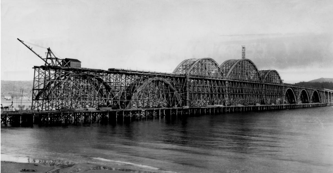
Big timber is marching across the bay, the Alsea Bay Bridge under construction in 1935.
