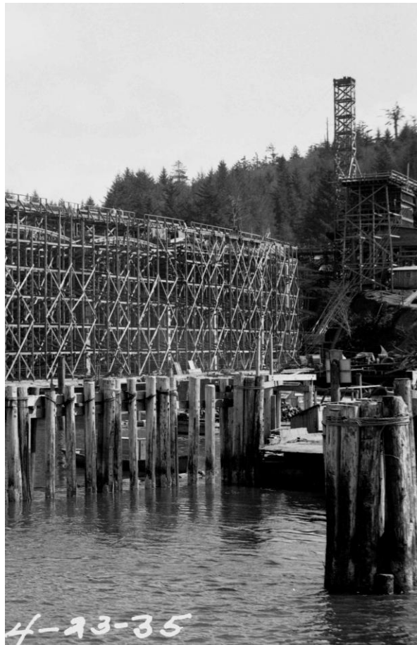
Wood forms for pouring concrete starting over the Siuslaw River.
