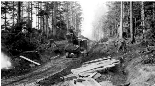
Early construction on the Oregon Coast Highway near Arch Cape.
