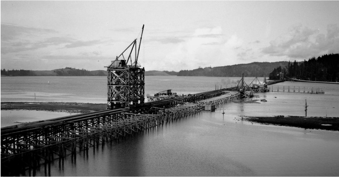
You are looking at the initial piling going in for the bridge over Coos Bay at North Bend in 1935.
