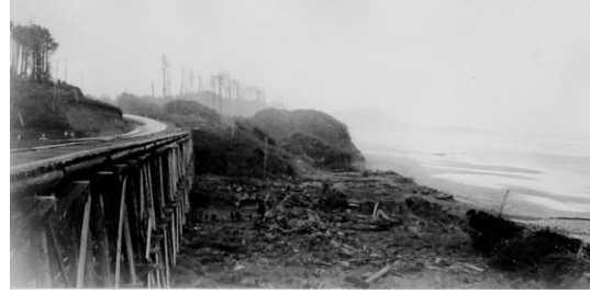
South bound on an early timber bridge over Moolach Creek near Lincoln City in the twenties.
