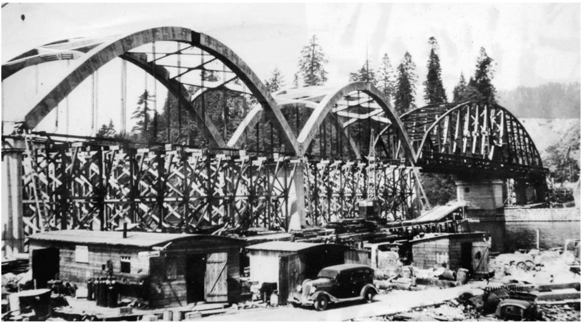
The Umpqua River Bridge under construction near Reedsport, Oregon in 1935.
